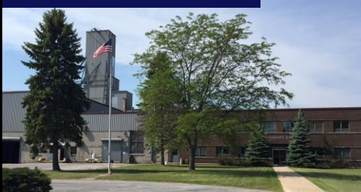
3,800 tpd shaft and major surface infrastructure
